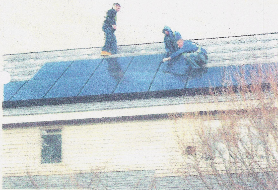
Jason Williams, left, electrician, and Matt Robichaud and Mike Richards, both apprentices, of New England Breeze Solar, install solar panels on a home on Cameron Road, as part of the Solarize Harvard program. COURTESY PHOTO
